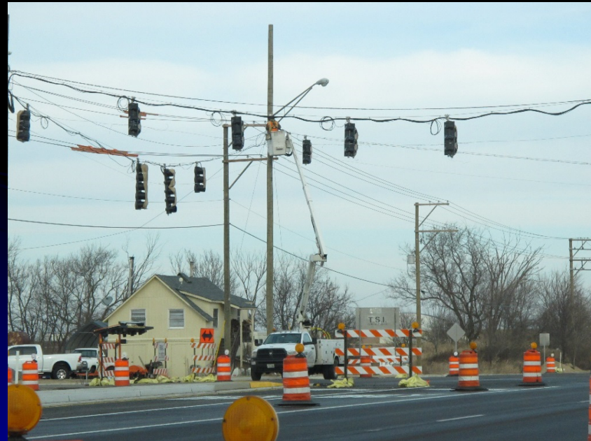
Landscaping crews button up some loose ends as electrical crews set signal heads and work on the controller box on the Longmeadow Parkway at Randall Road
